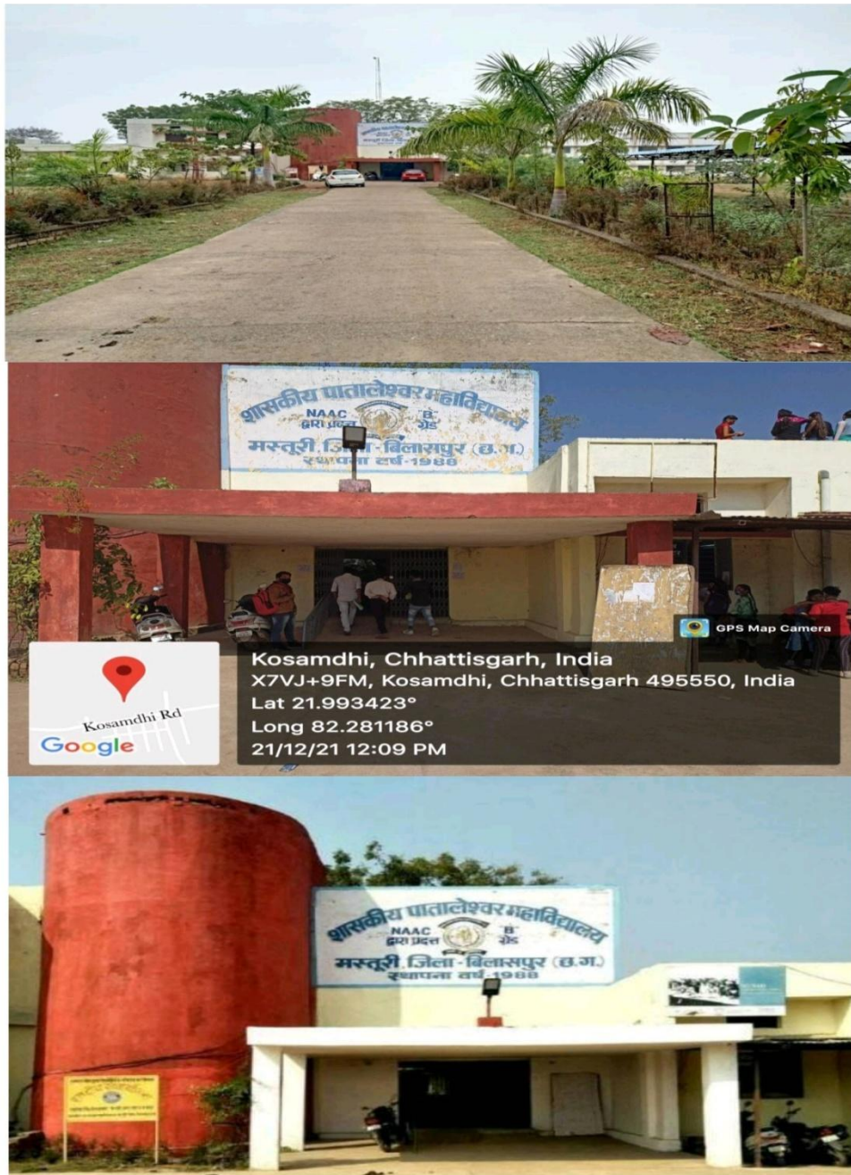
Fig . COLLEGE BUILDING
