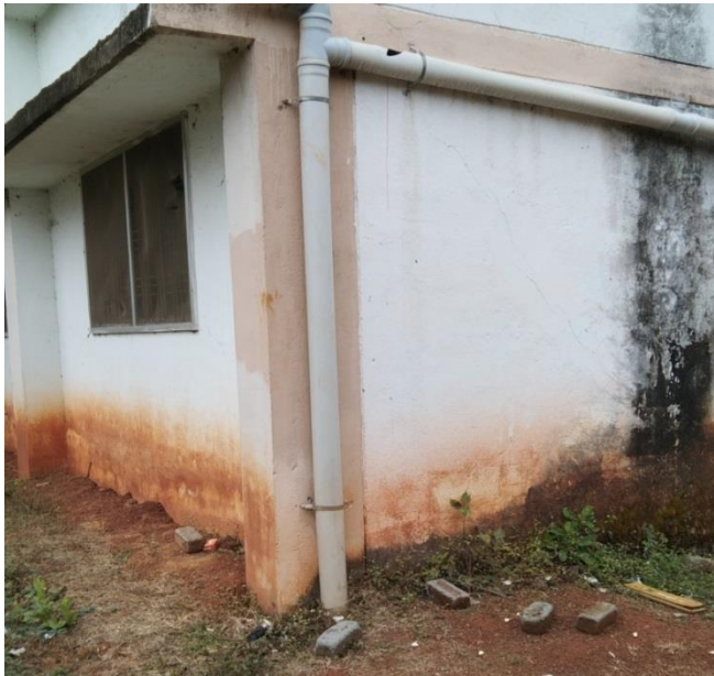
Fig. 19 Water Harvesting System
