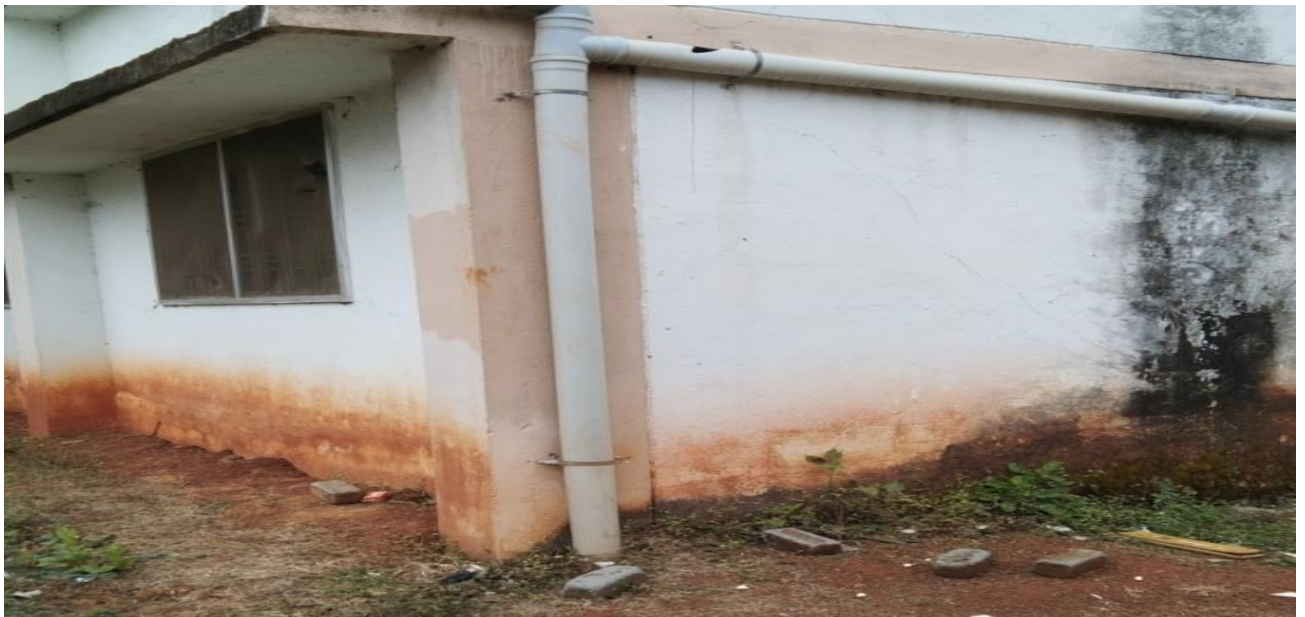
Fig. 14 Water harvesting system Showing the faunal diversity of the college
