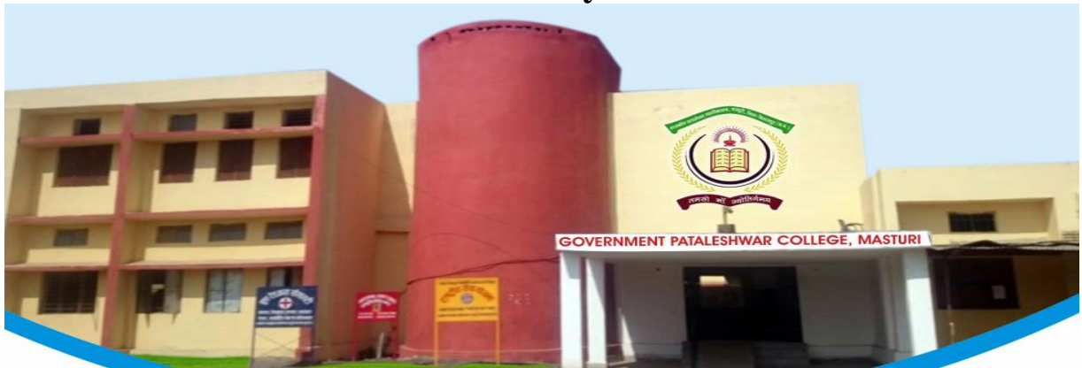
Fig. 1 Government Pataleshwar College, Masturi (Administrative Block)
