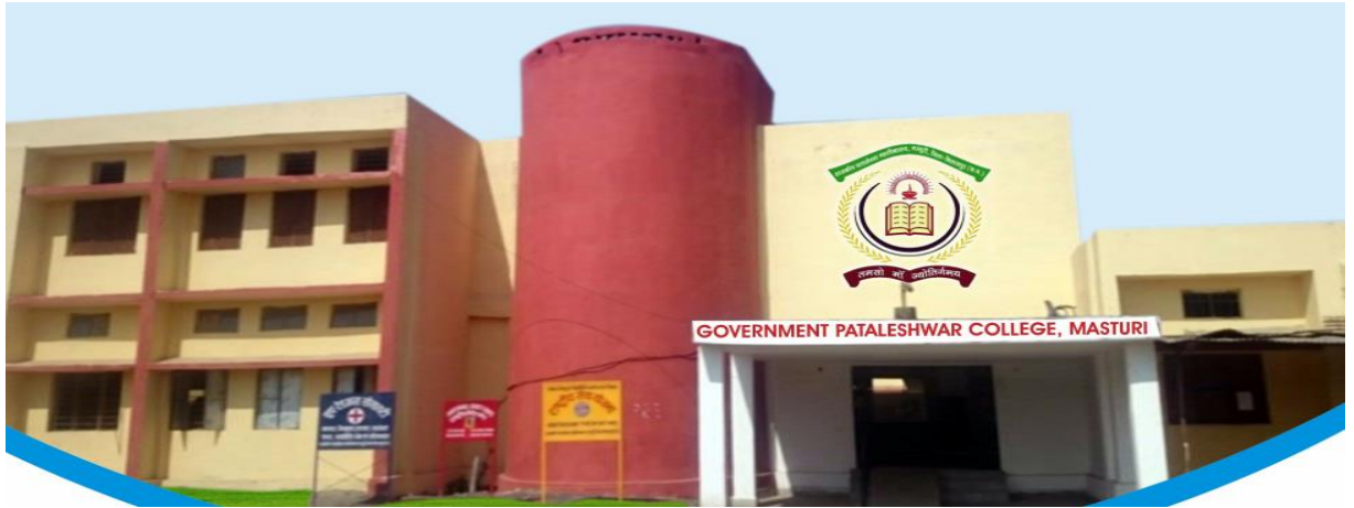
Fig. 1 Government Pataleshwar College, Masturi (Administrative Block)
