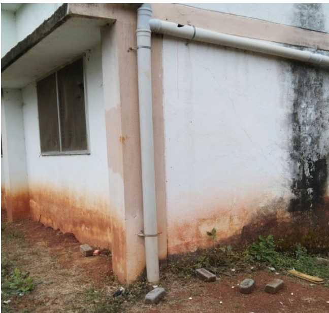
Fig. 16 Water harvesting System
