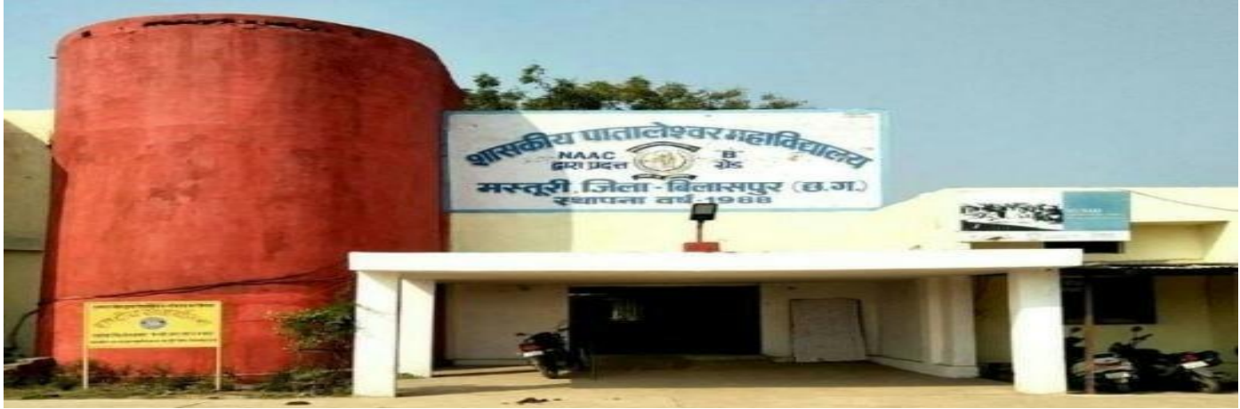
Fig. 1 Government Pataleshwar College, Masturi (Administrative Block)
